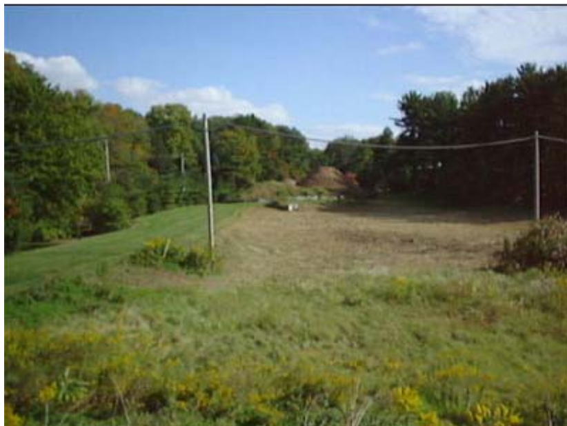
Figure 1.5: Original Detention Basin
