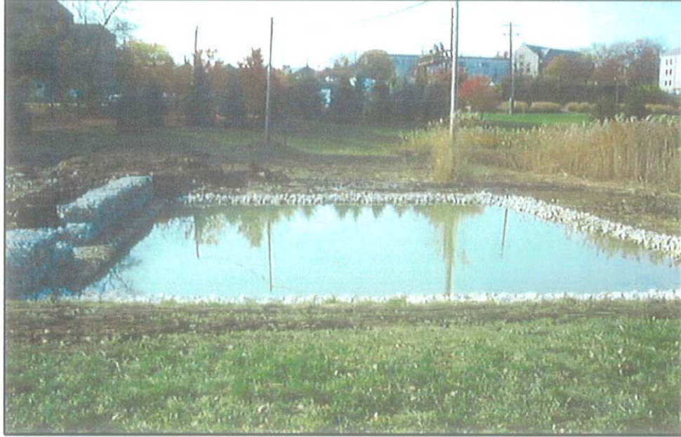
Figure 1.9: Sediment Forebay. The gabion weir is located on the left and controls the flow leaving the Sediment Forebay.
