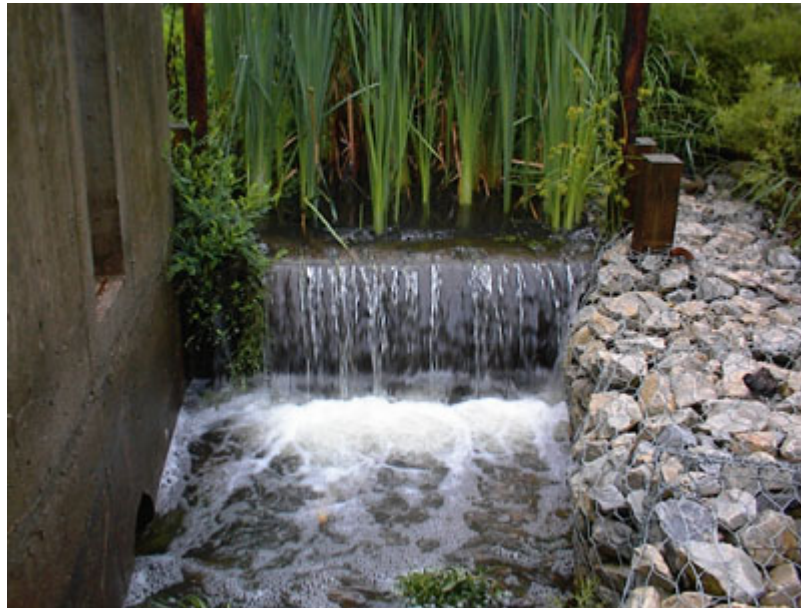
Figure 1.9: Sediment Forebay. The gabion weir is located on the left and controls the flow leaving the Sediment Forebay.
