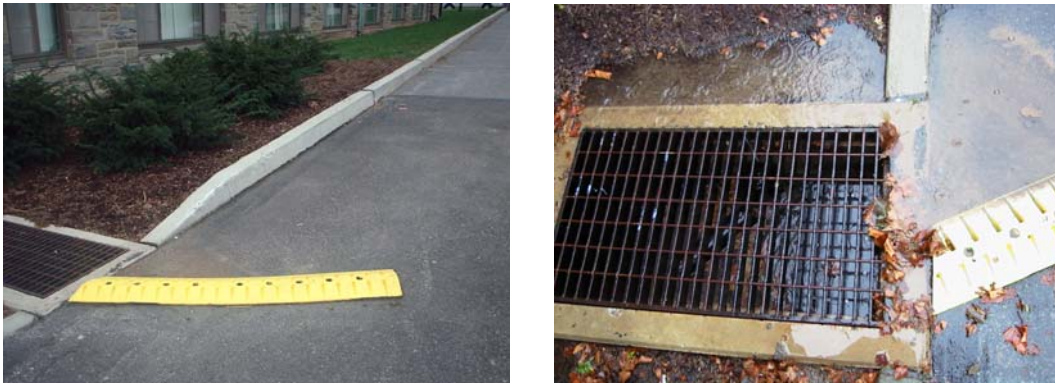
Figure 1.7 Speed Bump After Installation (left) and During a Storm (right)
