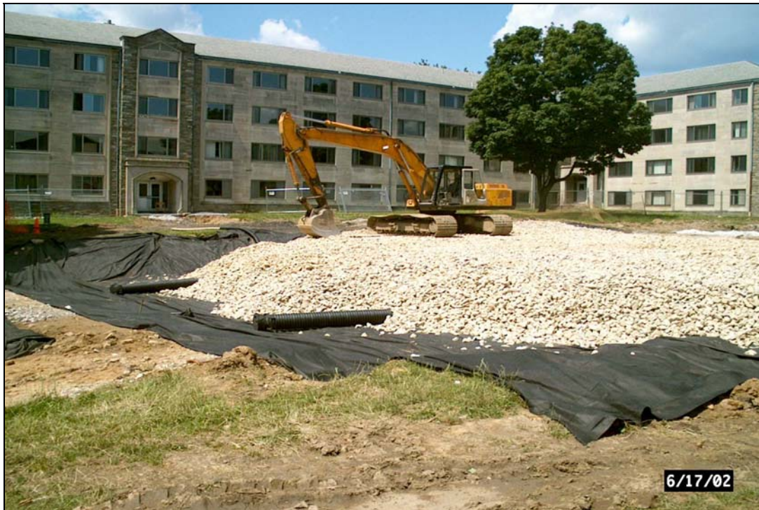
Figure 1.9 Middle Infiltration Bed Under Construction
