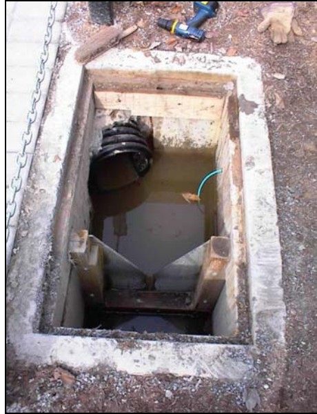
Figure 1.11 Weir Outlet Control Structure
