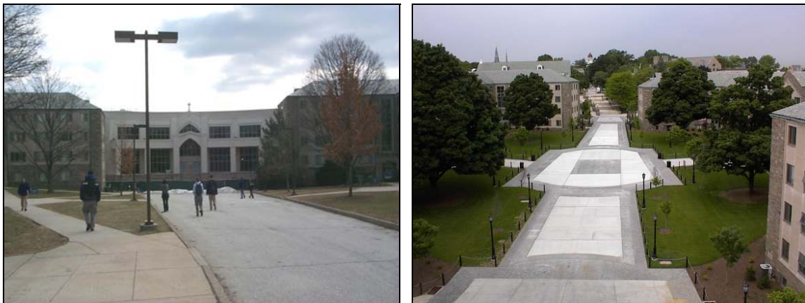
Figure 1.3 Pre (left) and Post (right) Construction Photograph of the Porous Concrete Site
